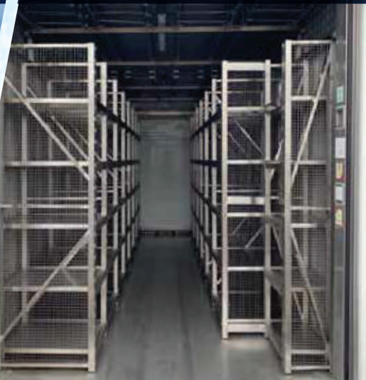
SHELVES AND RACKING
